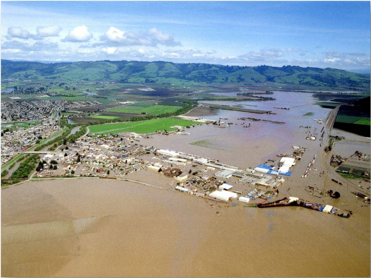
Figure 3. Flooding in town of Pajaro, 1995.
