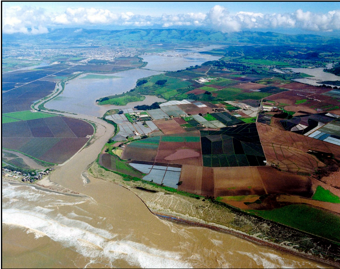
Figure 9: Flooding from Pajaro River in Monterey County, 1995
